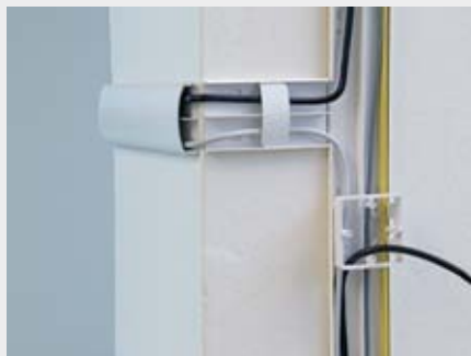
Installation of the elegant LE trunking system.
