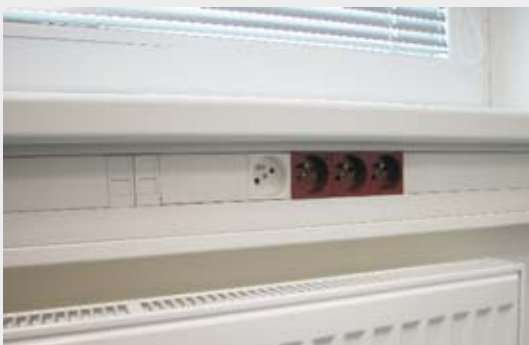
Example of installing the PK 120X55 D parapet trunking.
